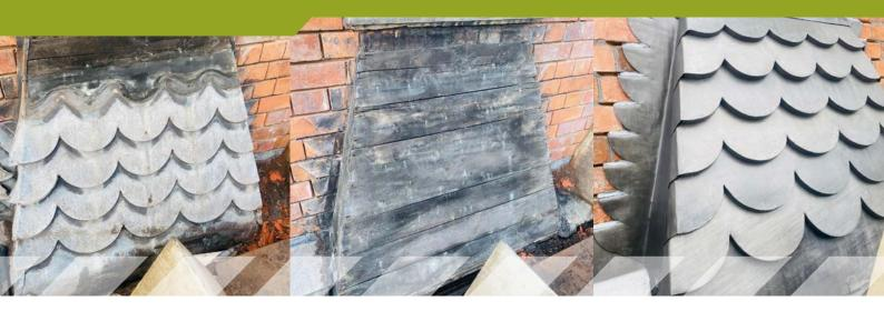
The project is set for completion later in 2024. A key part of the restoration involved the careful replacement of the slated roof, which NRA completed in just four weeks. Much of the original timber needed replacement, including bullnose detailing, to enhance the roof's durability while preserving its original design.
