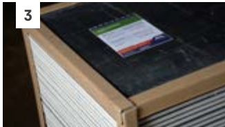
3 Each board is clearly labelled by location, weight, lead code and board type.
