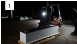
1 Boards are sorted onto pallets according to room and wall location.
