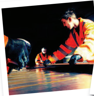
All lead-lined boards are purpose-made onsite
