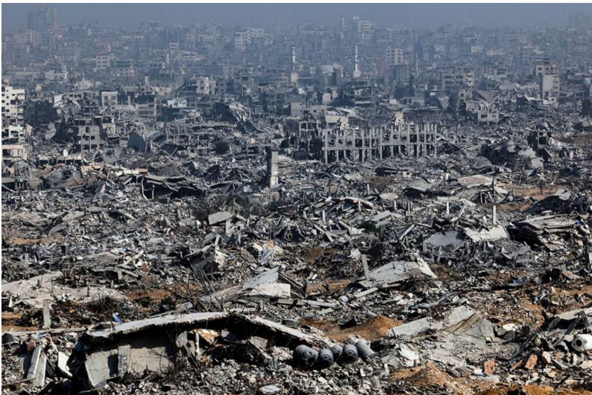
La Guaira, Venezuela - June 25, 2026: The city damaged in the aftermath of powerful earthquakes.
